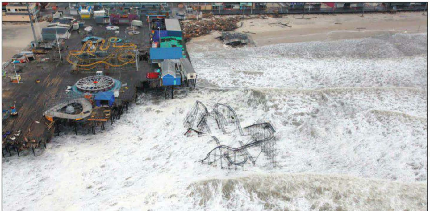
Photo B- Casino Pier at Seaside Heights in New Jersey's Ocean County, is a soggy mess in the aftermath of Hurricane Sandy. (Courtesy of Wikimedia Commons)
