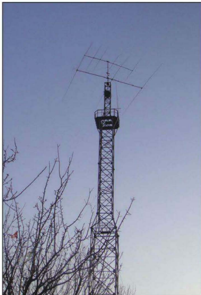
Photo E— Another one of B1Z's five towers. Each tower supports one or more monband Yagis.
