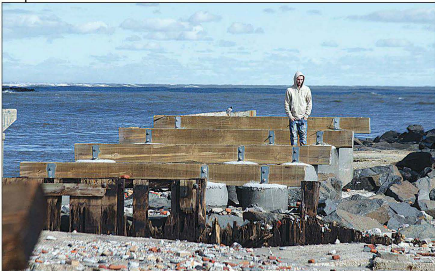
Like this portion of the historic boardwalk in Atlantic City, New Jersey, many cell phone sites were destroyed by the fierce winds of Hurricane Sandy. Amateur radio remains one form of communications that works “when all else fails.” (Photo by Liz Roll/FEMA)
